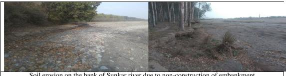
Soil erosion on the bank of Sunkar river due to non-construction of embankment (kms 1.650 to 5.100)
